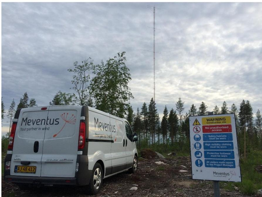
To date, we have installed and serviced over 70 masts in the Nordic and Central European region. The majority of these installations are in rough, mountainous and arctic terrain, including the recent installation of a 180m mast outfitted with over 30 sensors for a research project in Southern Sweden. Many of our masts are equipped with a Meventus power supply to power high consumption instrument heating (See our “Hybrid Power Systems” brochure for more information).
